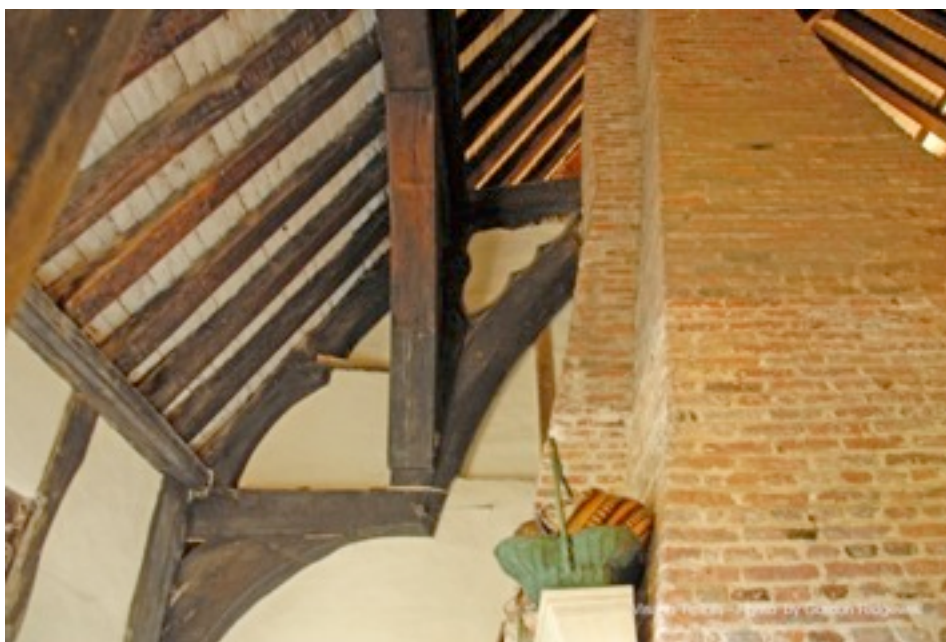
Massive scalloped edge hammerbeam
