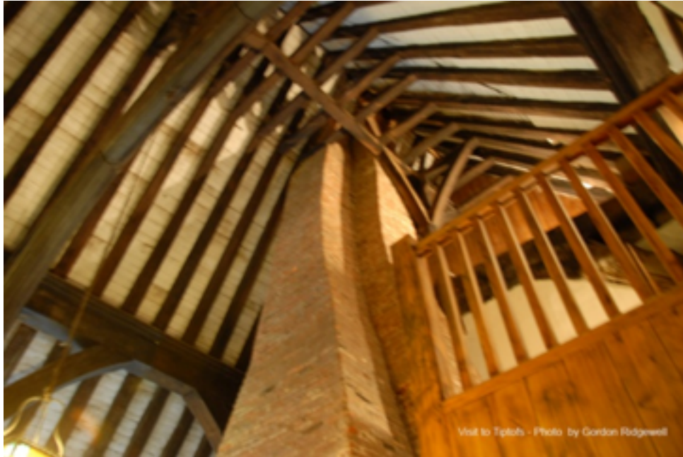
Exposed roof timbers surround the 16 th century chimney stack
