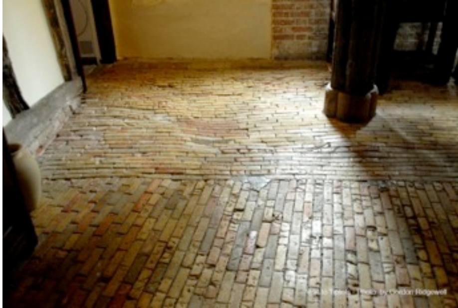
Brick floors support the timber frame and aisle pillars
