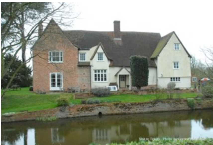
Rear view noting the steep roof
