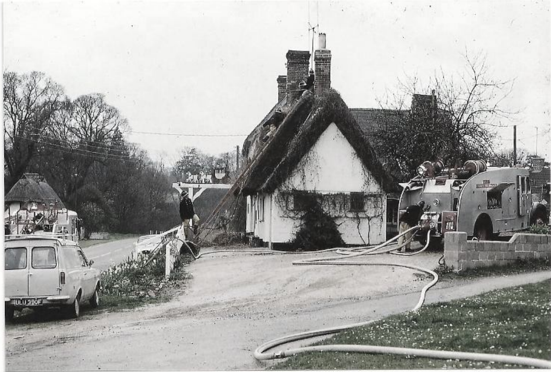
Newport Fire Brigade removing burning thatch from the roof in the 1960s.
